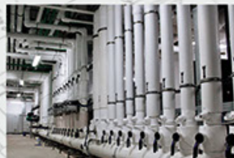
Pre-Insulated Manifolds and Pipes, Aqua-Plus Prins in 5* Hotel compound
